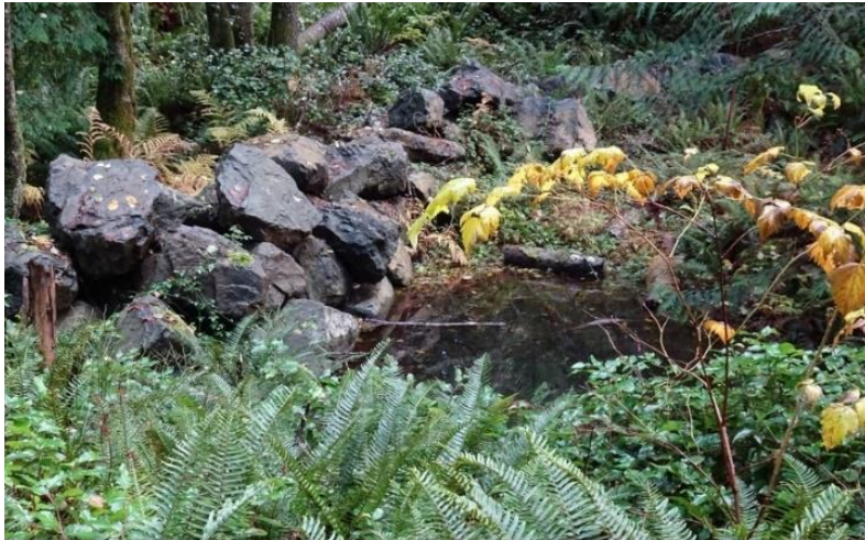
Boulders put down as "diffusers" to control water flow in the event of failure of the Morrell Lake dam (2021)
